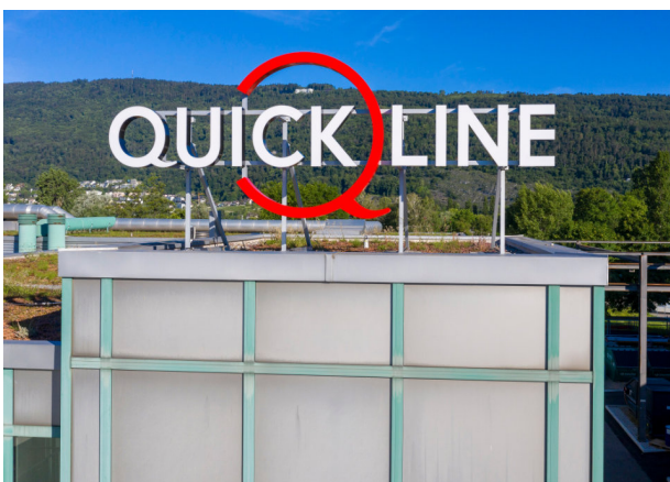
Illustration: outside view of the building Nidau (Source: Mediendownload@quickline.ch)
